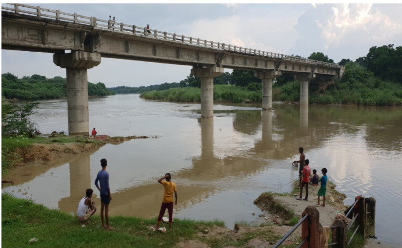
Bridge on River Sai
